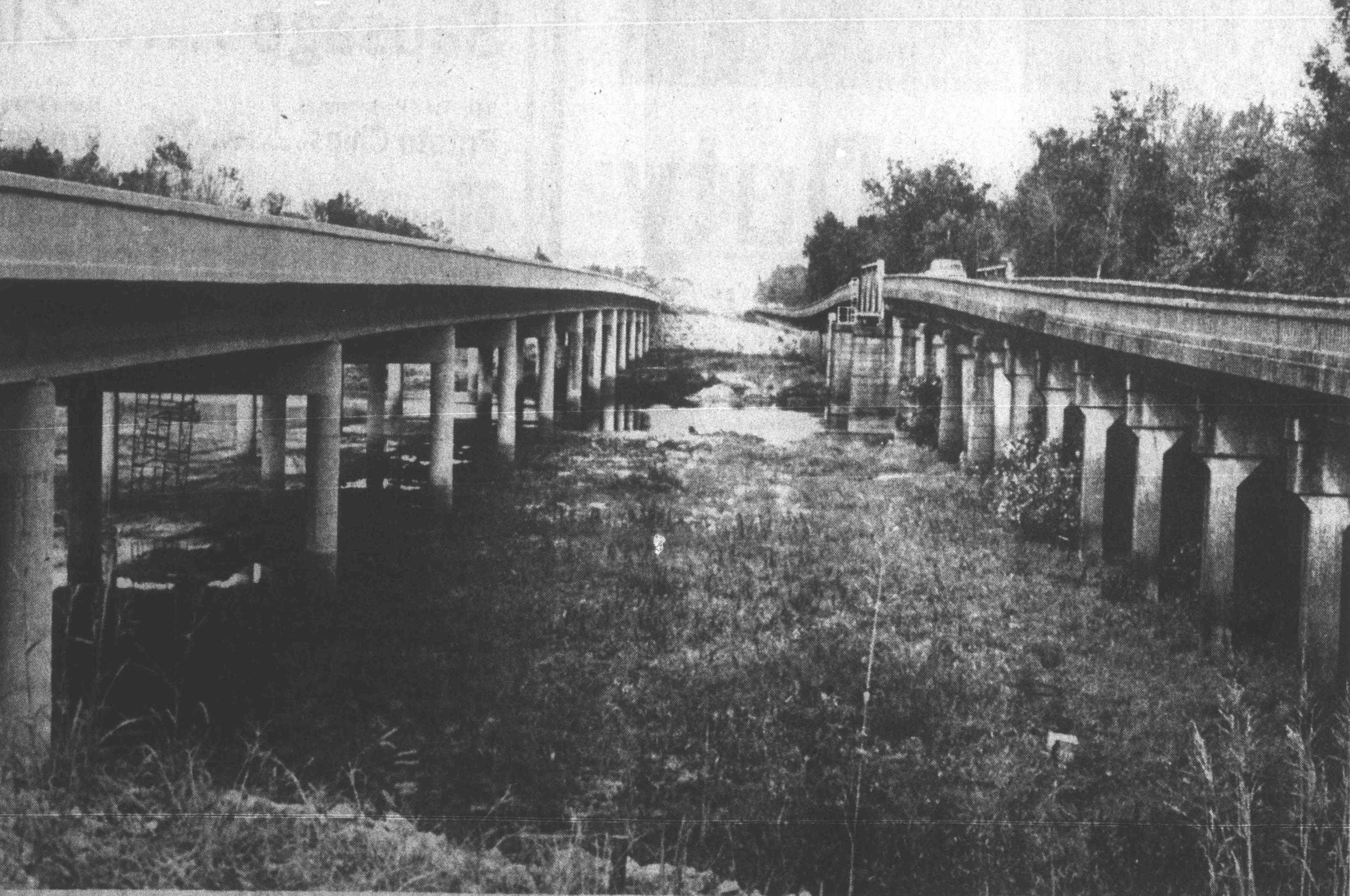
NEW SPAN ACROSS THE HATCHIE RIVER on Highway 51, between Henning and Covington, is scheduled to open Dec. 1st. The new bridge, at left above, four-lanes the highway from Memphis to Dyersburg, with a leg from Dyersburg to Troy still two-lane.
